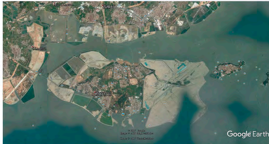
Xiamen New airport construction site
